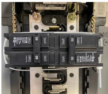
6 Reinstall breakers in spaces 5 & 6 once the breaker retainer is installed
