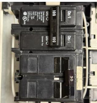
6 Reinstall breakers once the breaker retainer is installed
