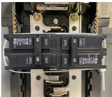
6 Temporarily remove the retainer and mark drill holes. Using the provided drill bit, drill through the back of the panel's rear cover. Once done, reattach the retainer and secure it with the **GREEN** self-tapping screws and apply the **NOTICE** sticker.
