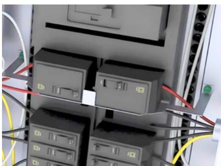
6 Temporarily remove the retainer and mark drill holes. Using the provided drill bit, drill through the back of the panel's rear cover. Once done, reattach the retainer and secure it with the **GREEN** self-tapping screws and apply the **NOTICE** sticker.
