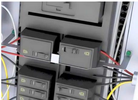
6 Reinstall breakers in spaces 5 & 6 once the breaker retainer is installed.
