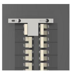
Set the **MAIN** and **GENERATOR** 9 breakers in the **OFF** positions and reattach the panel cover.
