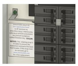
Drill through the holes in both the back plate and the panel cover. On the back side of the panel cover, file or scrape each hole to ensure proper grounding for the kit. The binding screw must make direct metal-to-metal contact with the back of the panel cover.
