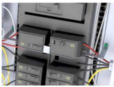
Temporarily remove the retainer and mark drill holes. Using the provided drill bit, drill through the back of the panel's rear cover. Once done, reattach the retainer and secure it with the GREEN self-tapping screws and apply the **NOTICE** sticker.
