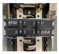
Temporarily remove the retainer and mark drill holes. Using the provided drill bit, drill through the back of the panel's rear cover. Once done, reattach the retainer and secure it with the **GREEN** self-tapping screws and apply the **NOTICE** sticker.
