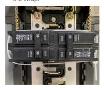
Temporarily remove the retainer and mark drill holes. Using the provided drill bit, drill through the back of the panel's rear cover. Once done, reattach the retainer and secure it with the **GREEN** self-tapping screws and apply the **NOTICE** sticker.
