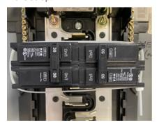
Temporarily remove the retainer and mark drill holes. Using the provided drill bit, drill through the back of the panel's rear cover. Once done, reattach the retainer and secure it with the **GREEN** self-tapping screws and apply the **NOTICE** sticker.
