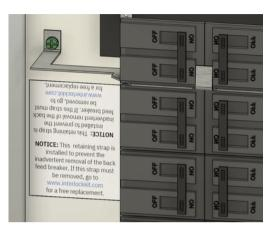
Drill through the holes in both the back plate and the panel cover. On the back side of the panel cover, file or scrape each hole to ensure proper grounding for the kit. The binding screw must make direct metal-to-metal contact with the back of the panel cover.
